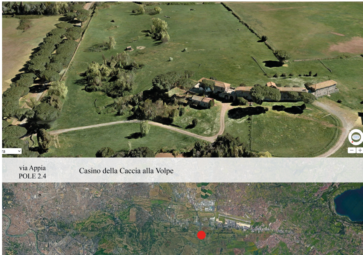
Fig. 5 Representative images of the pole of intervention 2.4 (PA-Appia Archive).
